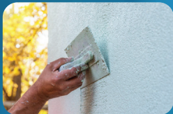
Exterior wall coatings
